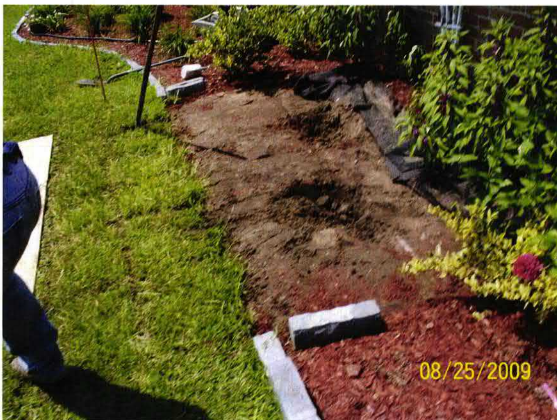
Picture 2: UST 1225Dove location prior to excavation and after removal of bedding.
