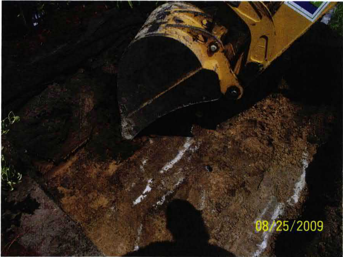
Picture 3: Removal of concrete on top of tank
